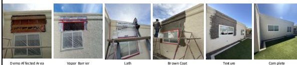
Demo Affected Area Vapor Barrier Lath Brown Coat Textured Corn plate
